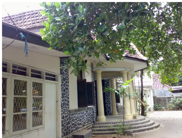
FIGURE (5). Façade of Bunga Rampai Restaurant Source: Agam Riadi Interior
