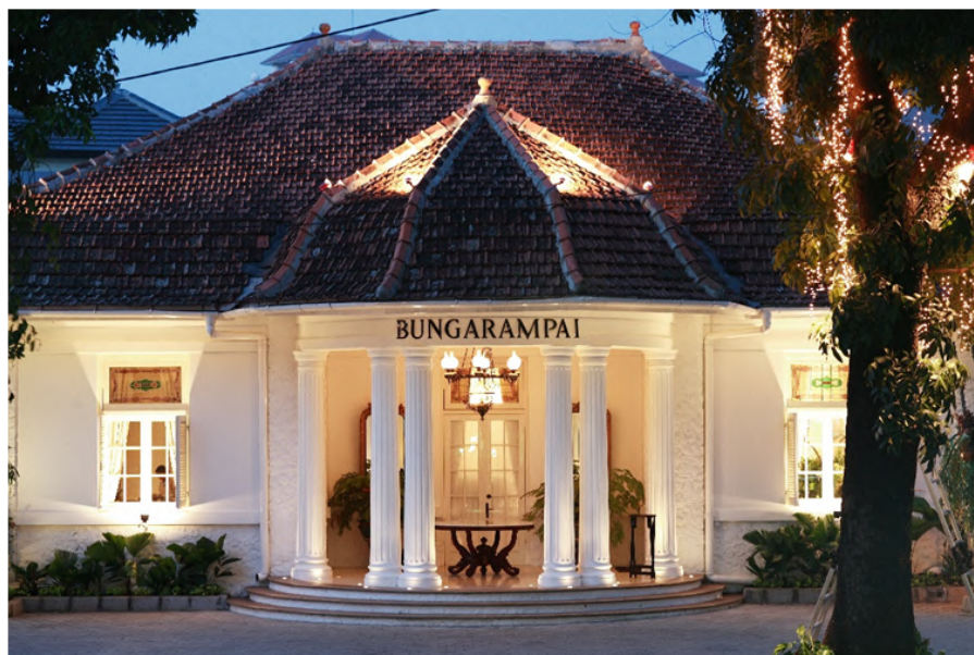
FIGURE (3). Façade of Bunga Rampai Restaurant Source: Agam Riadi Interior
